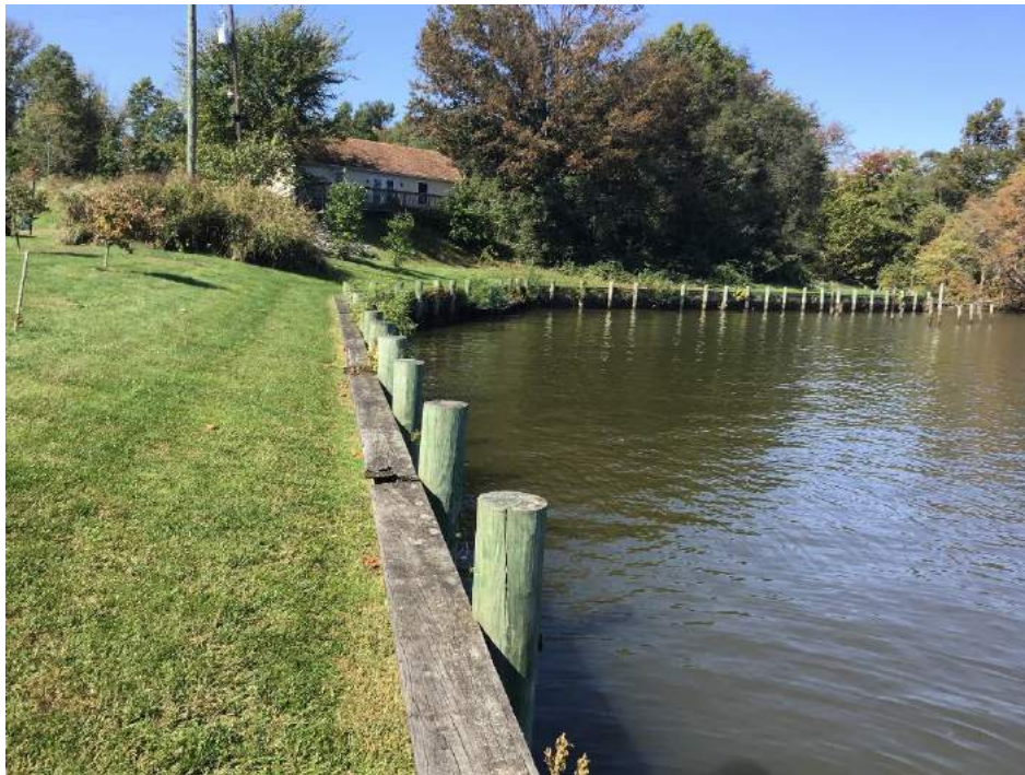
Photo 1: Existing bulkhead looking north towards the mouth of Peddlers Creek
