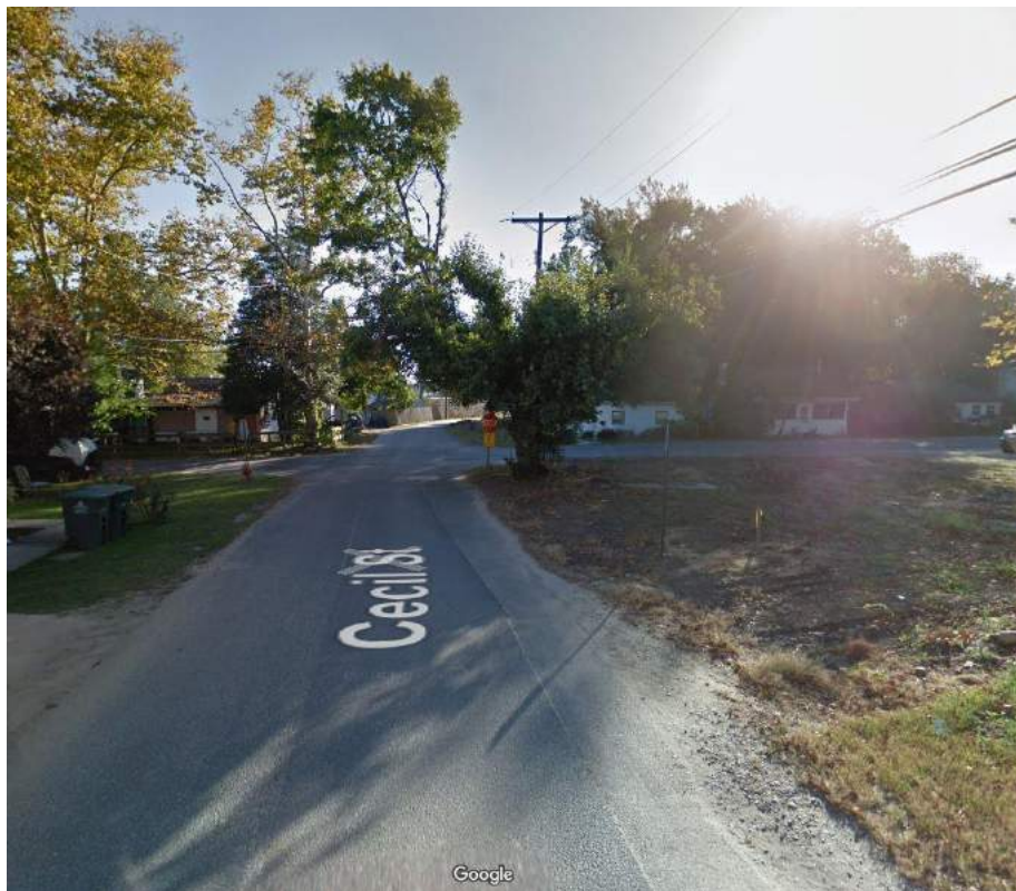
Photo 4: Cecil Street at Chesapeake Road intersection facing south
